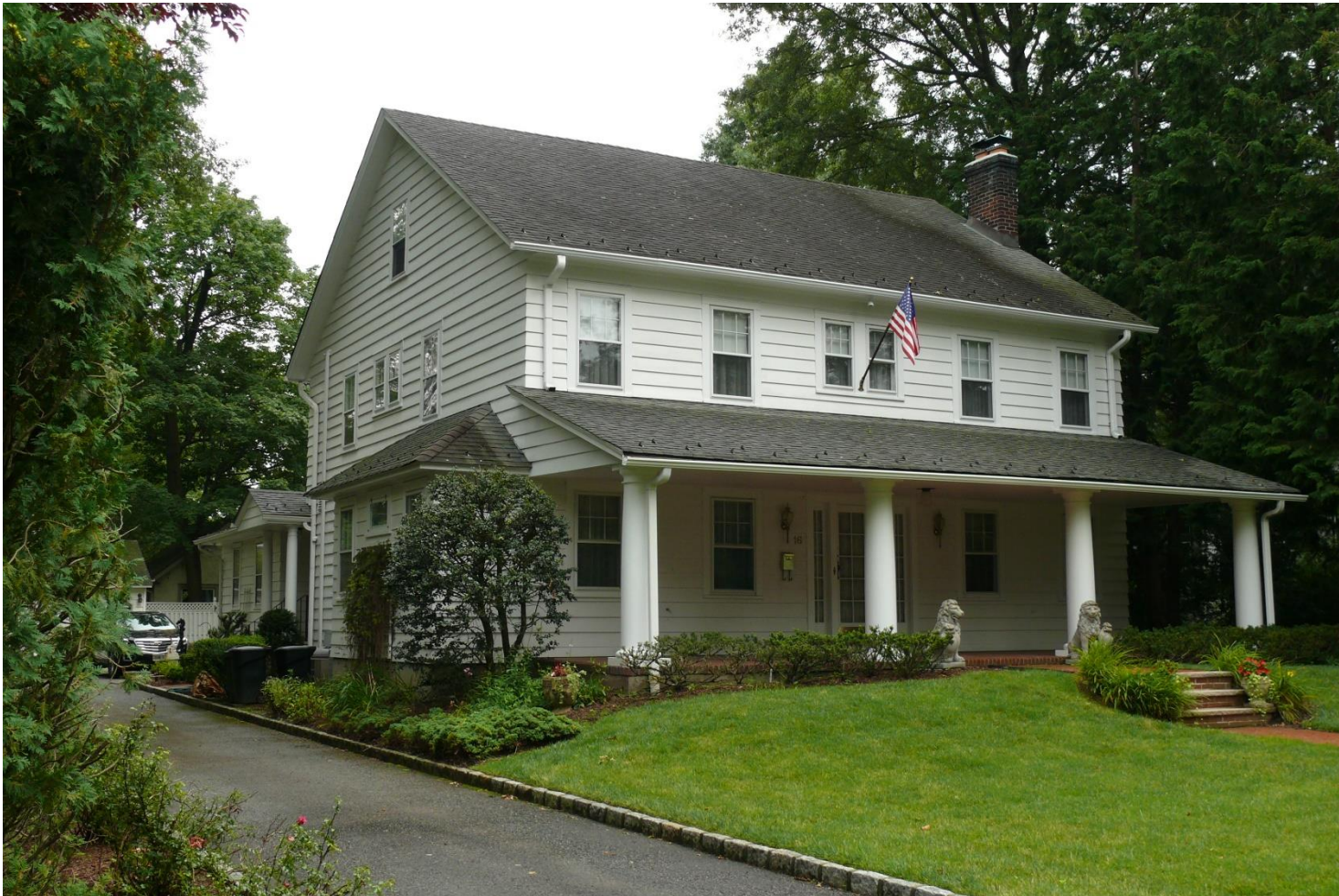
16 Parkside Street, 1927, Colonial Revival, Contributing
