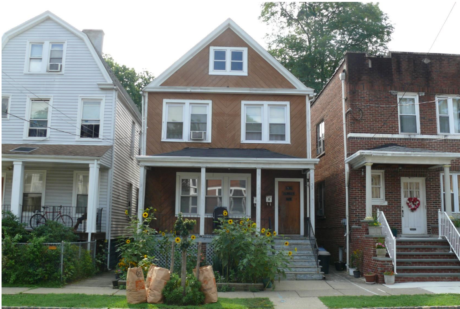
29 Wheeler Street: 1910, Vernacular, Contributing
