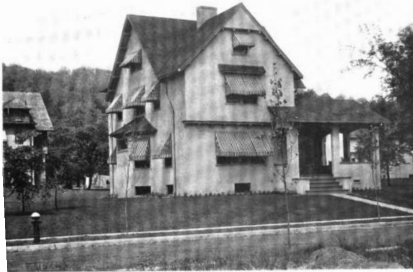
Figure 2 Mr. Lemkau's house is built of stucco, tinted a natural silver gray color
